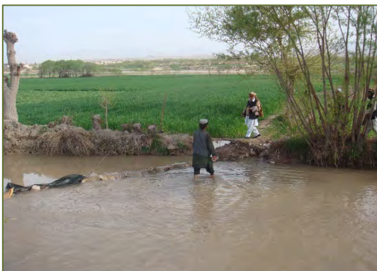
A view of selected water divider for construction in Charamgar canal
